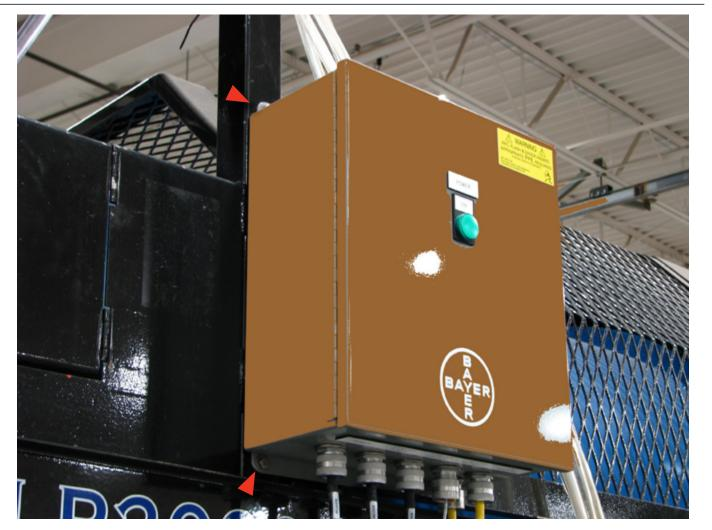
**JUNCTION BOX Step 1:** Use factory-supplied hardware and fasten the Junction Box to the Treater Frame, as shown above.
